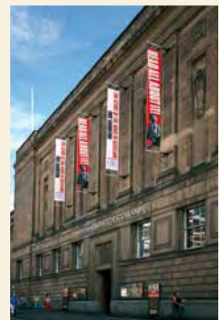
NLS on George IV Bridge
