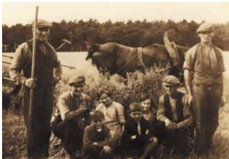
The Blythe family and farm workers, 1929. One of 6,000 items being digitised under the Resources for Learning in Scotland programme.
