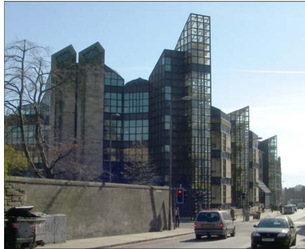
Figure 1: The Causewayside building of the National Library of Scotland, viewed from the north west.
